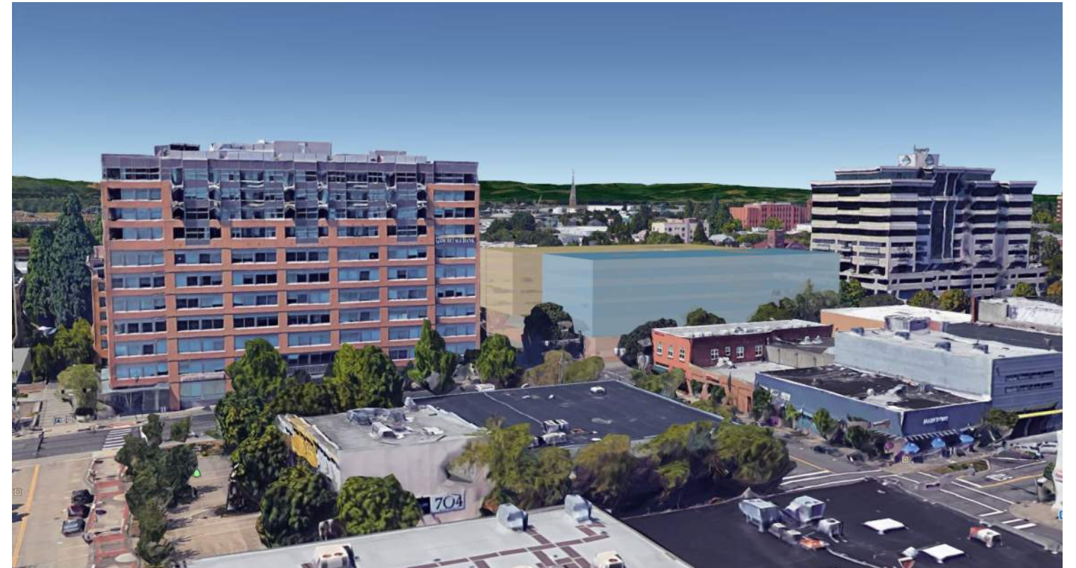
Looking North West
