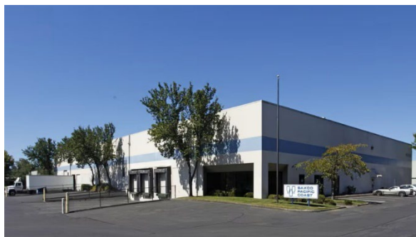
Example of Existing Warehouse in Vancouver, WA (70 KSF)
