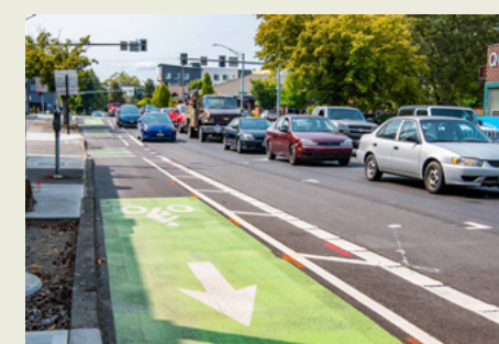
Vertical separation allows trucks and vulnerable users to co-exist. Photo: City of Vancouver
