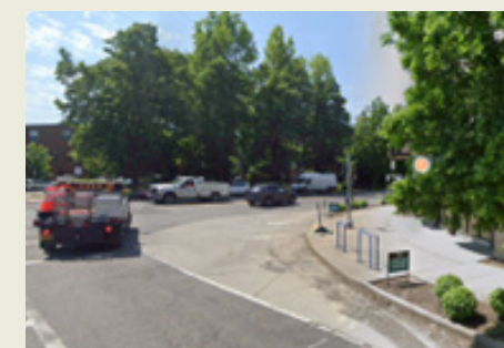
Mountable corners slow down passenger vehicles but can be mounted by trucks. Photo: Google Street View
